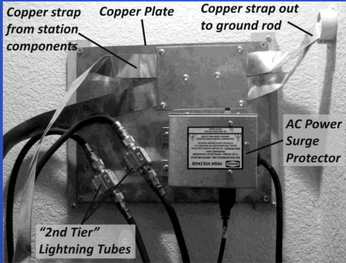
*An example wall-mounted single point ground panel with a second set of in-line coaxial lightning protectors and AC surge protector ground-mounted to panel, as well as ground straps from station component chassis.*
